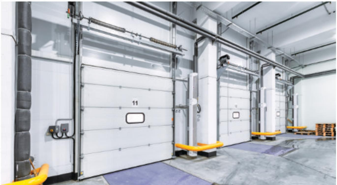
The GfA Elektromaten drive is mounted on a drive shaft mounted to the lintel. Lateral locking with a microswitch can be used (additional equipment table).
